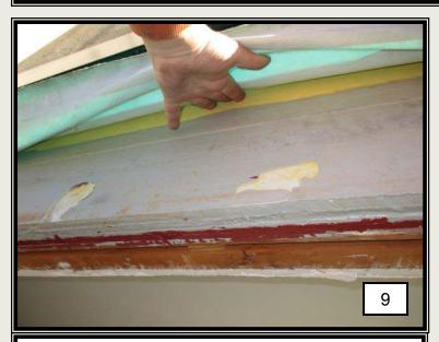
The Wet-Flash membrane is applied 9 inches above, and two inches into the rough opening of the Dens-Glass sheathing. No staining was observed on the exterior sheathing above the window opening.
