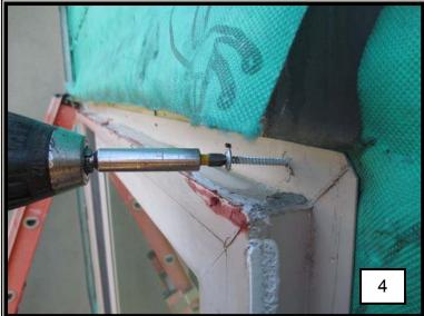
Mechanical fasters that secure the window were found to be corrosion free upon removal. The Vapro-Shield Weather Resistant Barrier was observed in good condition.
