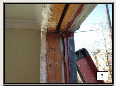
The BEI Wet-Flash is maintaining excellent adhesion to the wood substrate at the head and jambs of the rough opening.
