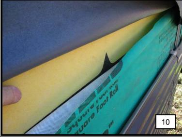
The Dens-glass exterior sheathing below the Sureflash at the sill of the opening was noted to be in as new condition. No deterioration or staining was observed on the face of the Dens-Glass.
