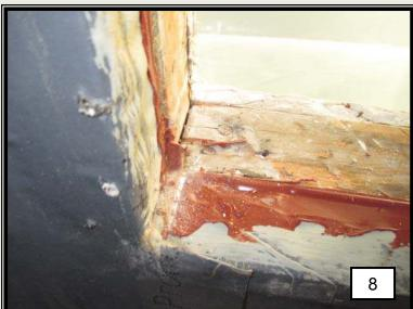
The Sure-Flash at the sill of the window is fully embedded into the Wet-Flash liquid applied membrane. No signs of water intrusion were visible at the framing of the rough opening.
