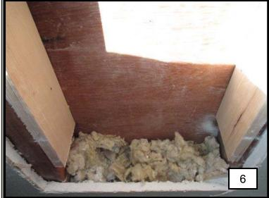
No staining was observed on the inboard side of the sheathing or the framing members and the insulation was noted clean and dry.
