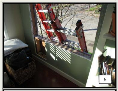
A cutout in the wallboard was made to observe the conditions in the wall cavity below the windows rough opening.
